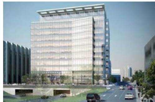
Downtown Medical Mixed Use Building Currently Being Built at 100 College Street
