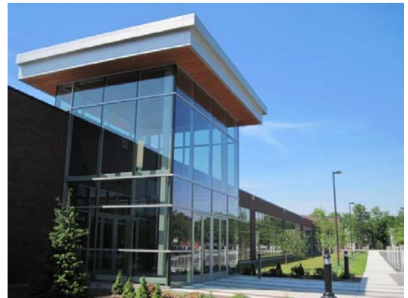
The newly built 245,000 sf office center on the historic Winchester Repeating Arms gun factory site at Science Park in Newhallville neighborhood. This building is now home to Yale's administrative offices, a print shop, and other offices
