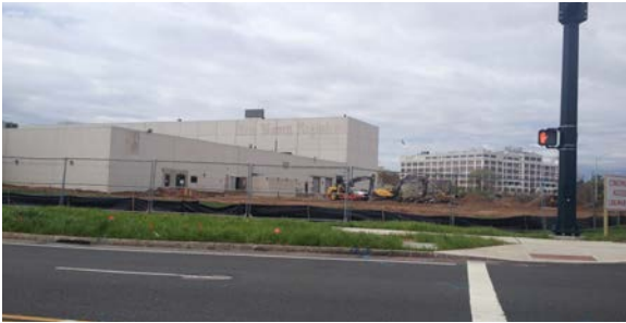
Construction is already underway to convert the former New Haven Register building at 40 Long Wharf Drive to a 200,000 square foot Jordan’s Furniture store featuring both retail and family entertainment opportunities.
