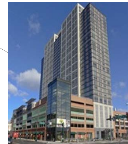
Downtown Residential Mixed Use Building at 360 State Street
