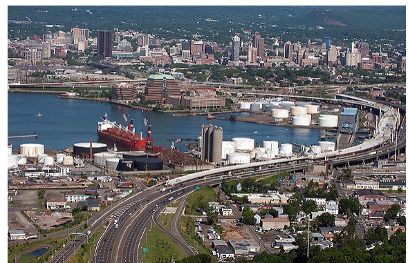
New Haven harbor is a regional distribution center for petroleum products, as well as the export of scrap metal.
