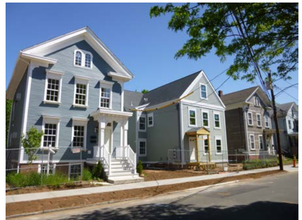
Recent residential rehabilitation on Putnam Street maintains the traditional character of the city’s housing stock.
