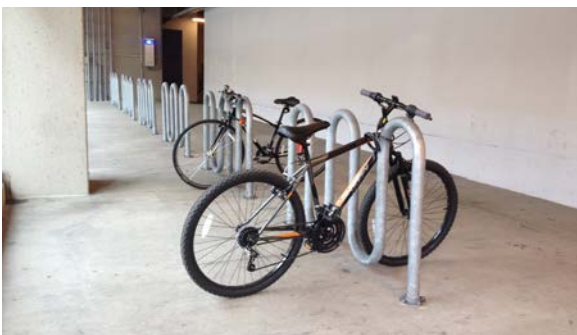
A secure indoor bicycle parking area was included in the construction program of the new downtown campus for Gateway Community College.
